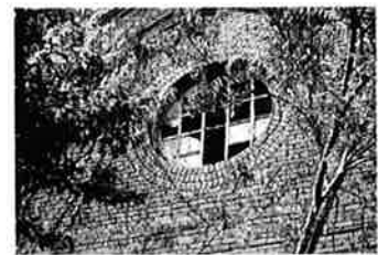
写真7・円形窓 (Paint shop)
